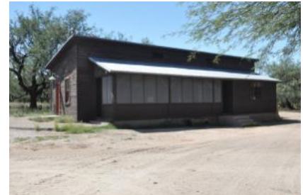
The Bunkhouse gets a screened-in addition
